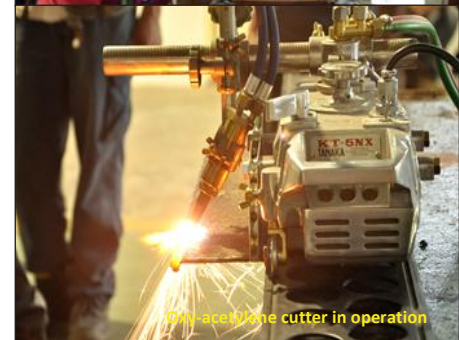
Welding Qualification Test in progress
