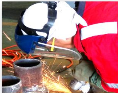
Grinding Work In Progress
